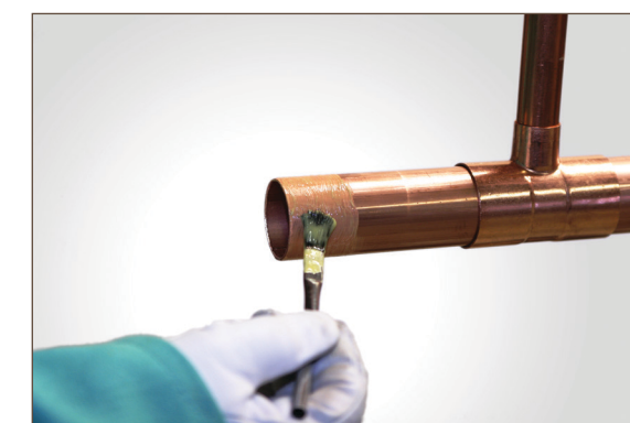
Figure 7.9. Fluxing: Tube
