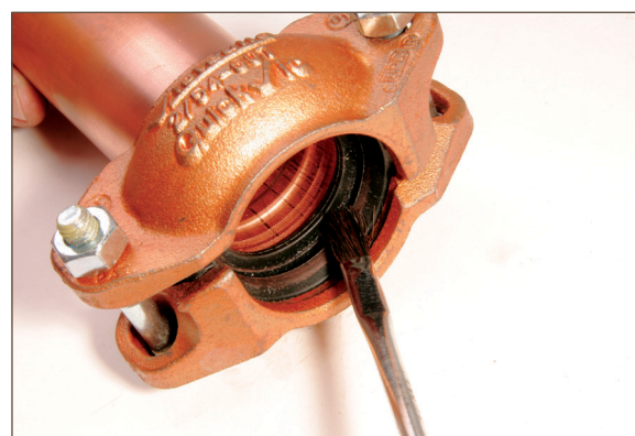
Figure 10.8. Applying lubrication to gasket
