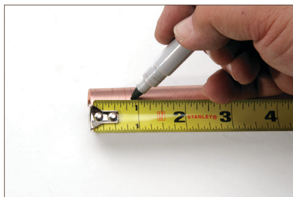
Figure 11.12. Measuring depth of insertion
