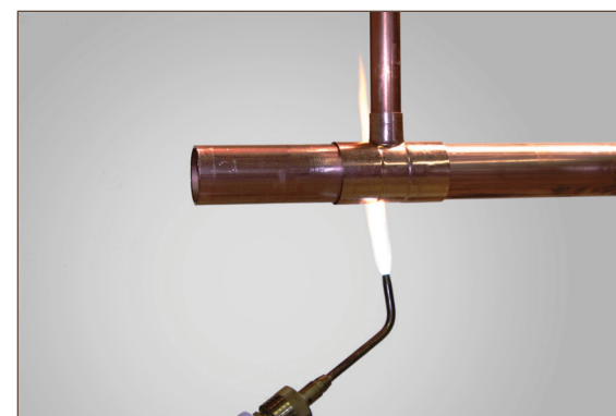
Figure 7.14. Preheating Fitting
