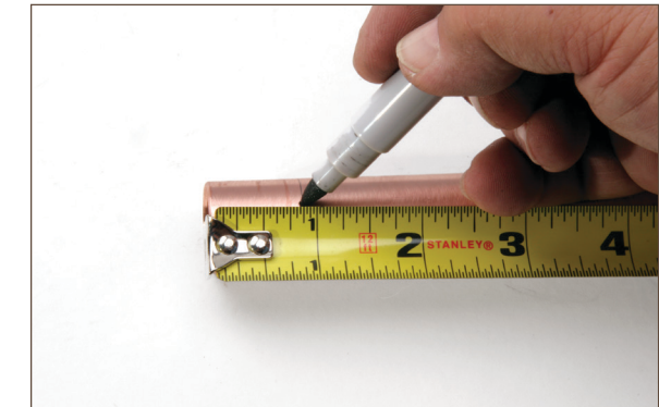
Figure 12.10. Making insertion depth
