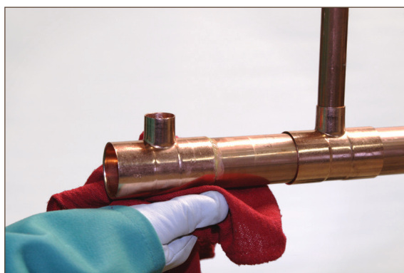
Figure 7.12. Removing Excess Flux
