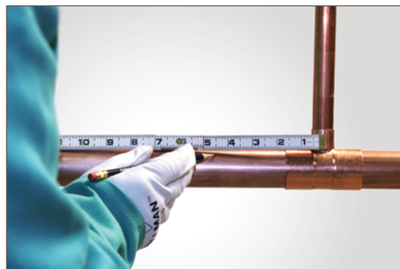
Figure 7.1. Measuring
