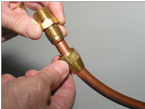
Figure 9.1. Flare Fitting/Flared Joint During Assembly
