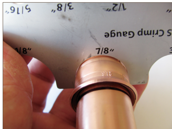
Figure 11.22. Correctly crimped fitting
