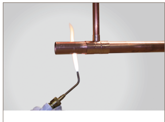
Figure 7.13. Preheating Tube
