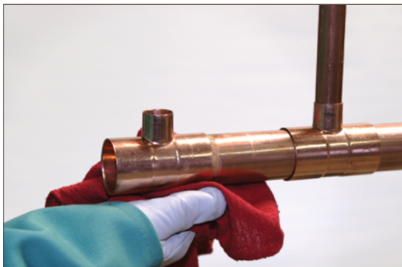
Figure 7.12. Removing Excess Flux
