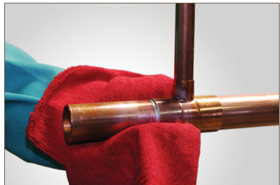
Figure 7.17. Cleaning
