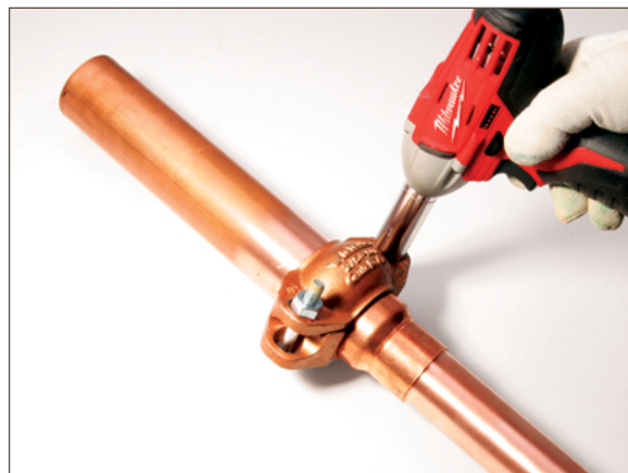
Figure 10.11. Tightening the clamp
