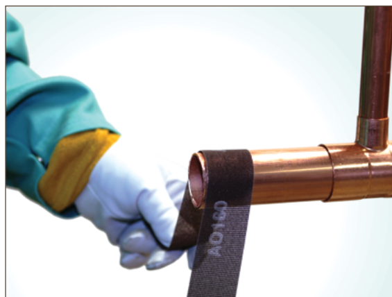
Figure 7.6. Cleaning: Sand Cloth
