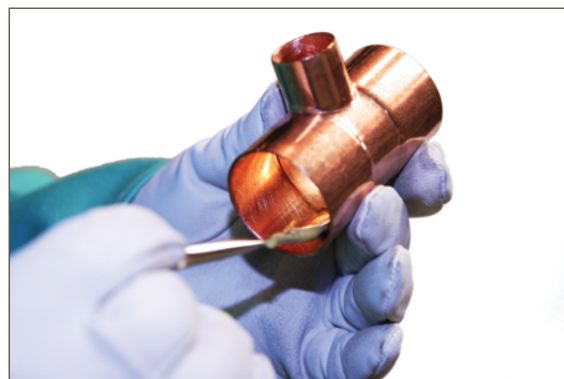
Figure 7.10. Fluxing: Fitting
