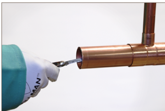
Figure 7.4. Reaming: Pocket Knife
