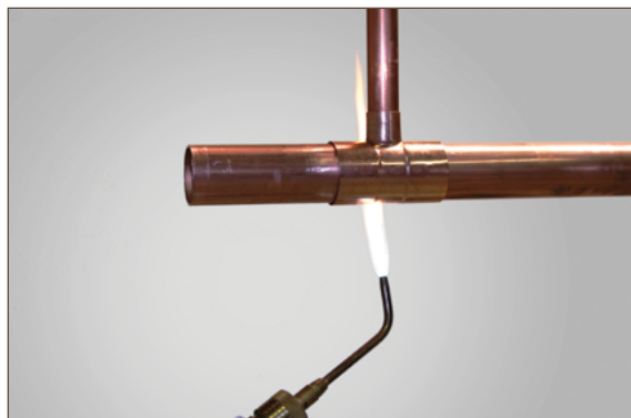
Figure 7.14. Preheating Fitting
