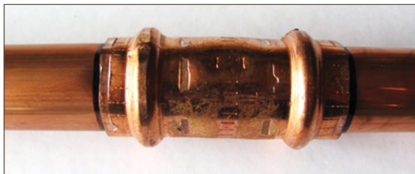
Figure 11.16. Completed installation of a press-connect joint
