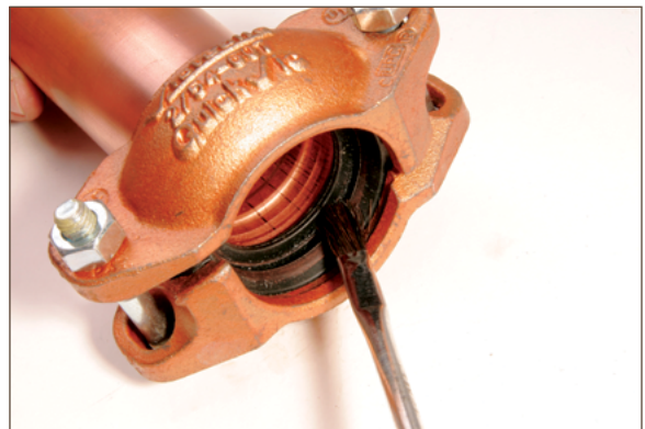
Figure 10.8. Applying lubrication to gasket
