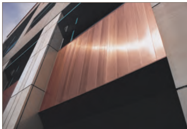
Figure 3.3A. The Anchor Center office building in Scottsdale, Arizona, chose to boast its location in the Copper State by preserving the natural color of freshly milled copper sheet with a clear coating. Due to sun and heat, the finish requires reapplication every few years to maintain its pristine look.
