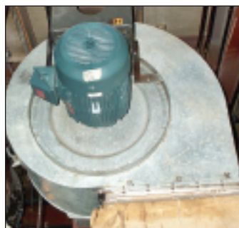
Figure 1. A 20-hp NEMA Premium motor drives a blower at Kodak Park. According to MotorMaster+, the motor saves the company 4,200 kWh and $315 per year compared with rewinding the standard-efficiency motor it replaced. This one small motor reduces annual carbon dioxide emissions by more than 5,400 pounds per year. Payback time for the new motor was only 1.1 years.
